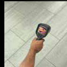
Check floorheating for leaks
