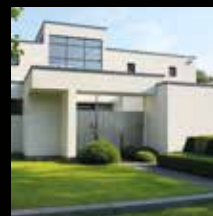
Find insulation problems
